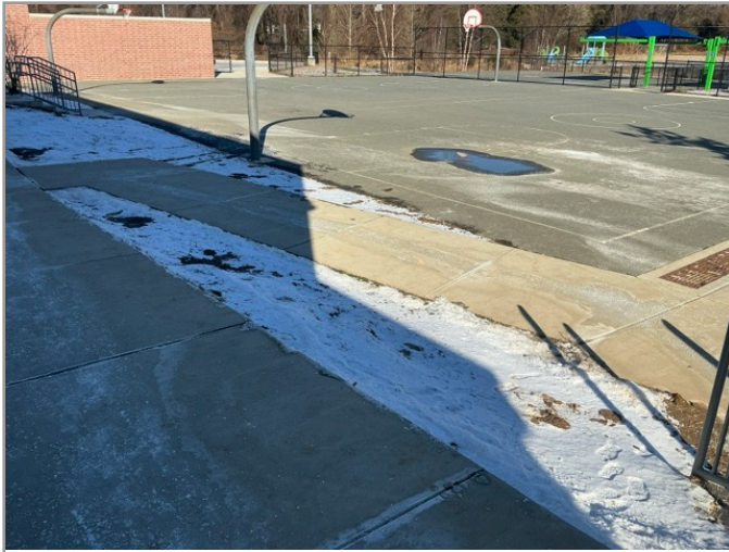
ACCESSIBLE ROUTE TO PLAYGROUND
