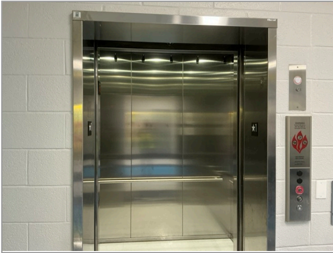
LOBBY LOOKING AT CABS (WITH DOORS OPEN)
