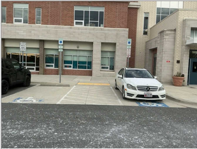
OVERVIEW OF ACCESSIBLE PARKING AREA
