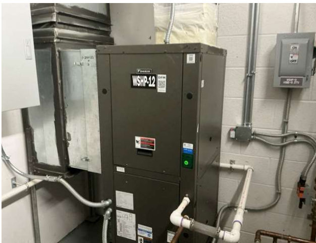
17 - WATER-SOURCE HEAT PUMP
